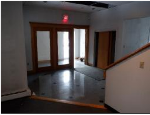
Interior, As-Is – 1st floor, entry and vestibule, looking NE
