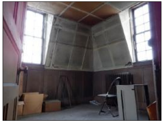
Interior, As-Is - attic, looking NE
