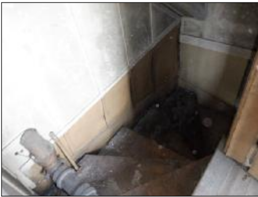
Interior, As-Is - attic, stairs
