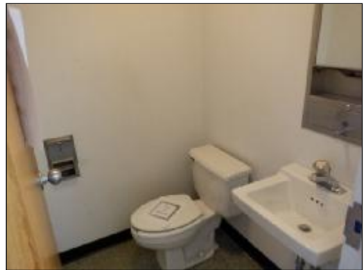
Interior, As-Is – 1st floor, 2-fixture bath
