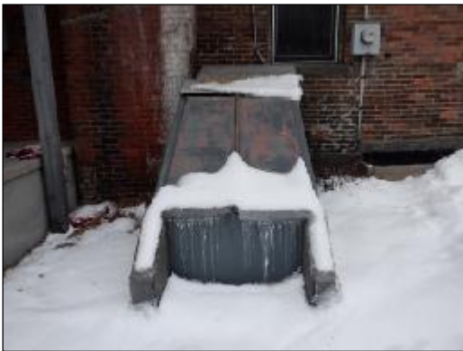
Exterior, As-Is – bulkhead access to basement
