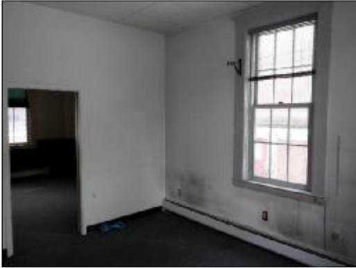
Interior, As-Is – 1st floor, office
