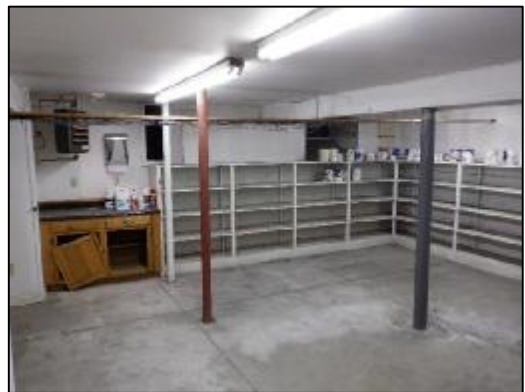
Interior, As-Is - basement, looking SW
