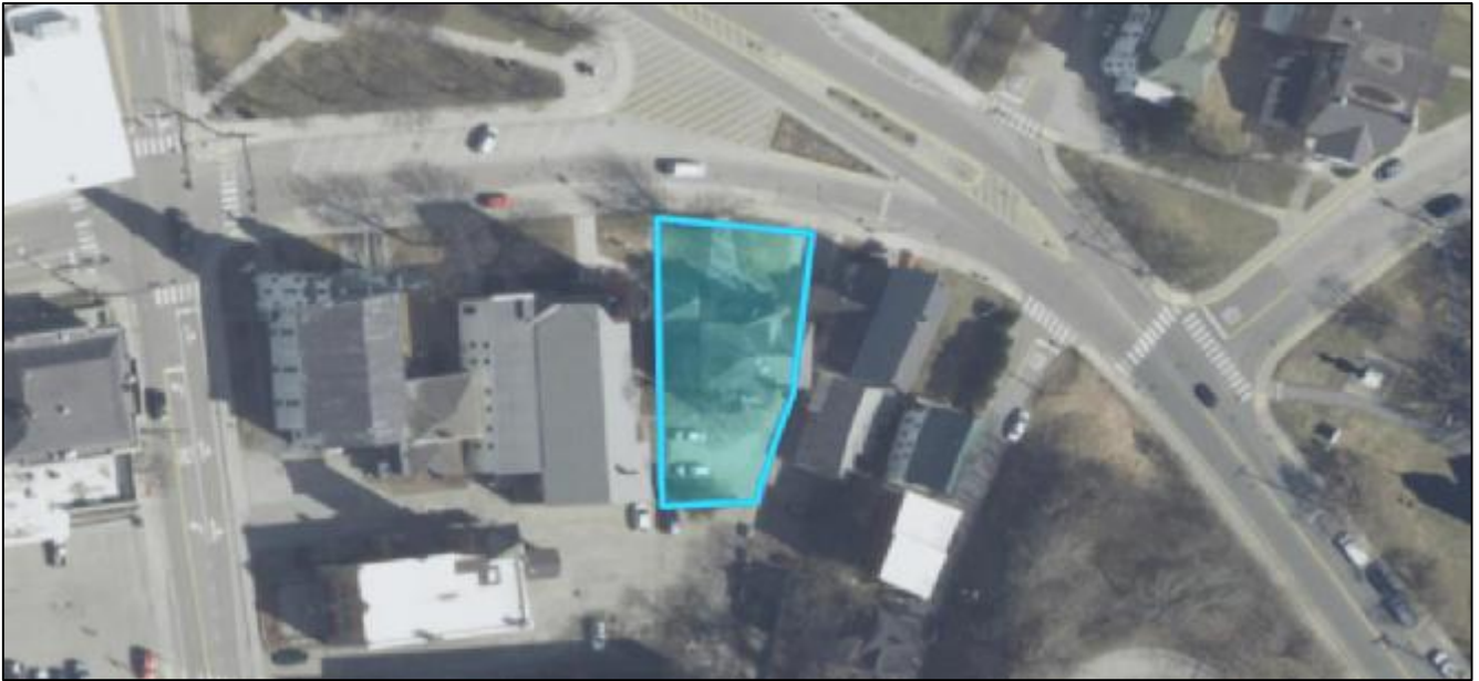
Aerial Photograph – approximate parcel boundaries highlighted
