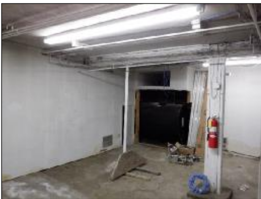
Interior, As-Is - basement, looking E
